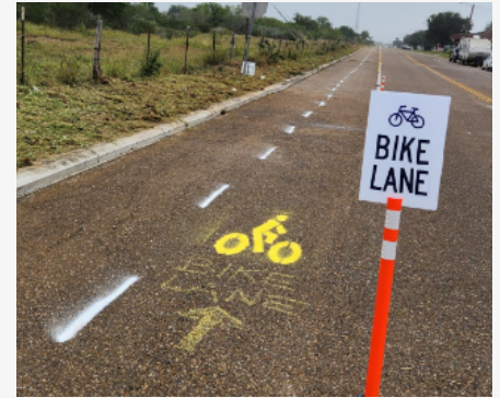
A pop-up bike/ped lane is installed along a roadway that connects two areas the town
